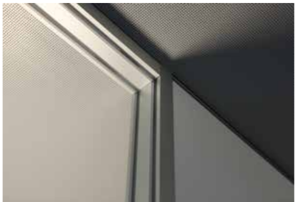
Double glass to solid panel integration
